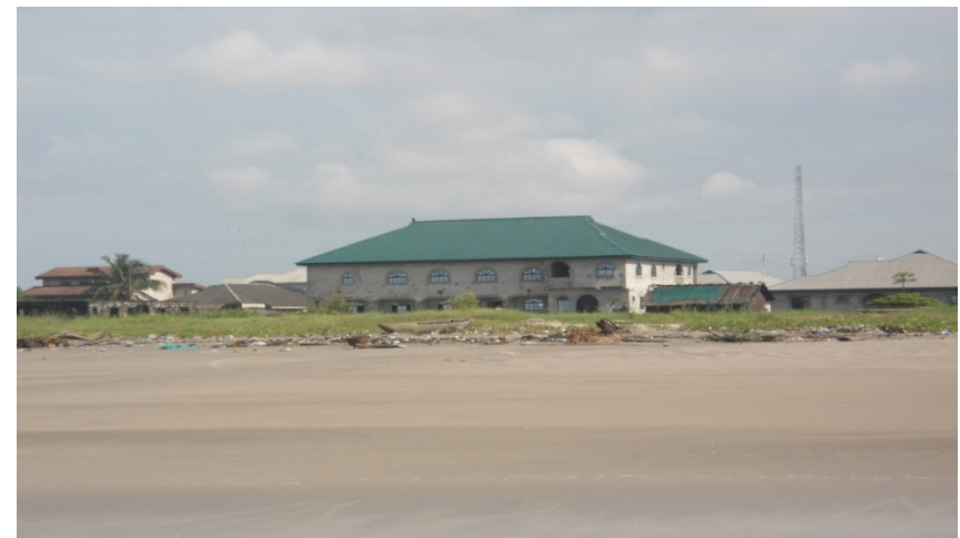
Plate 8: Foreshore- Downdrift Station 2
