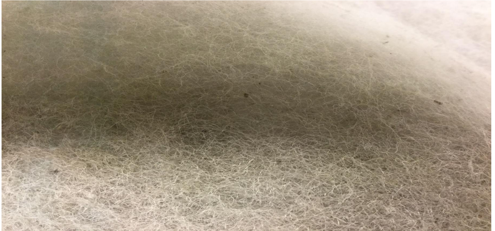
Air condition duct dibeer
