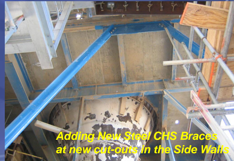
Adding New Steel CHS Braces at new cut-outs in the Side Walls
