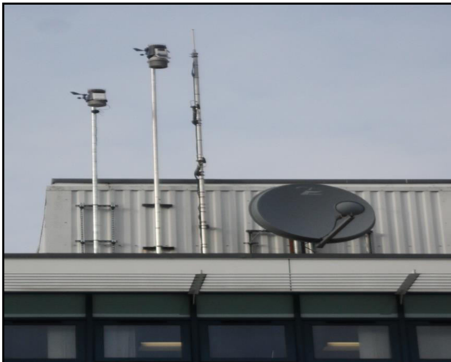
Facilities at Pontypridd South Wales
