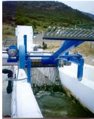
Automatic cleaning system (scraper)
