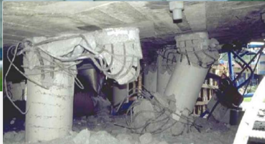
Storage tanks of Liquid Oxygen at Habas plant after the strong event of Itzmit (1999)
