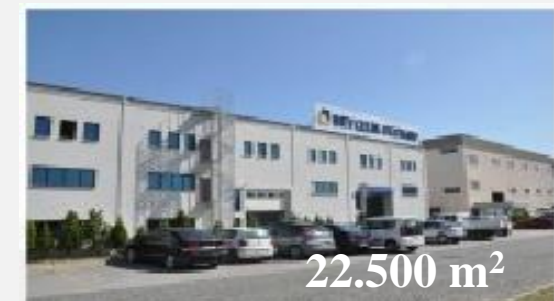
ASSEMBLY PLANT & STEEL CENTER
