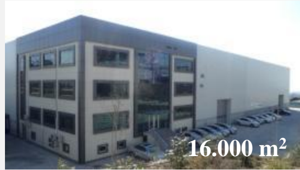
GEBZE CHASSIS PLANT
