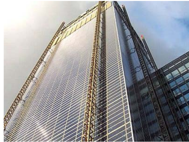
Solar Tower (Manchester, UK)
